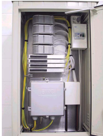
NHF System fiber node hub
