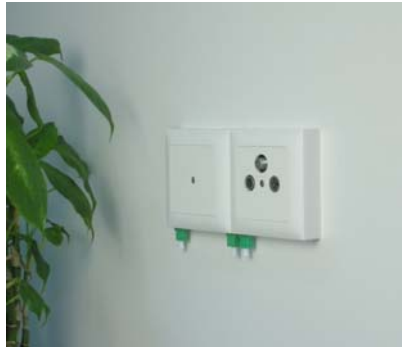
FTTH-Fiberdose (Micro Node NHP-0007)
